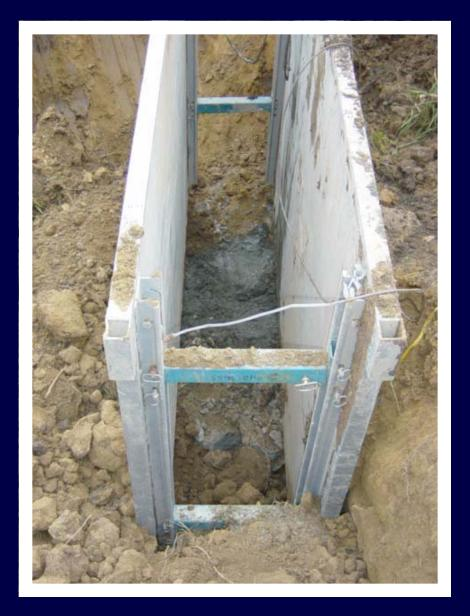
Set up of trench box on the primary acid waste line to gain access for plugging with concrete
