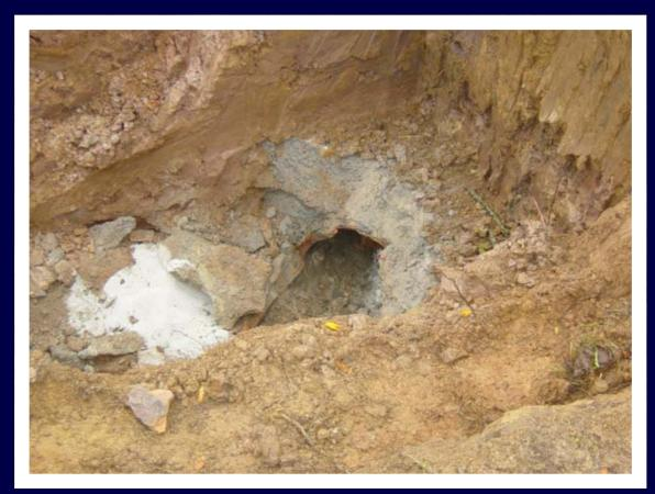
Opening of acid waste line prior to plugging with concrete
